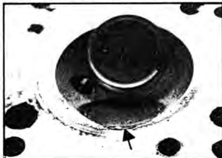
The exhaust seat also on No. 1 was fitted badly as well. Note the gap (arrowed) between the seat and the head, presumably where someone had tried to force the old seat out.
