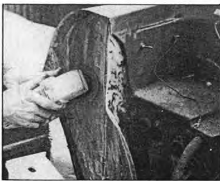
All bonding surfaces must be thoroughly prepared. Use the grinderette here or anything to abrade the surface well. Note master cylinders and hand brake cable have been removed.
