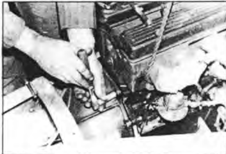
Bolting engine to gearbox.
